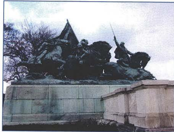
According to the U.S. National Park Service, green streaks are evidence of acid rain's effects. Photo from NPS
